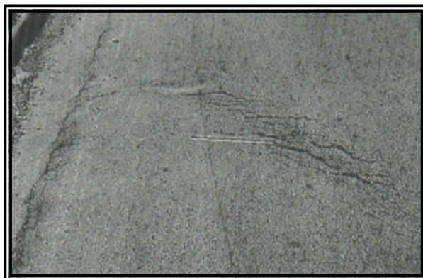
Figura 55: Grieta parabólica: severidad media. A photograph showing a wider, more irregular crack on a dark, textured surface. The crack is more pronounced and has some branching. A small white object is placed next to it for scale.
